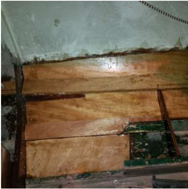
Fig 14: Aft Cabin Repairs
