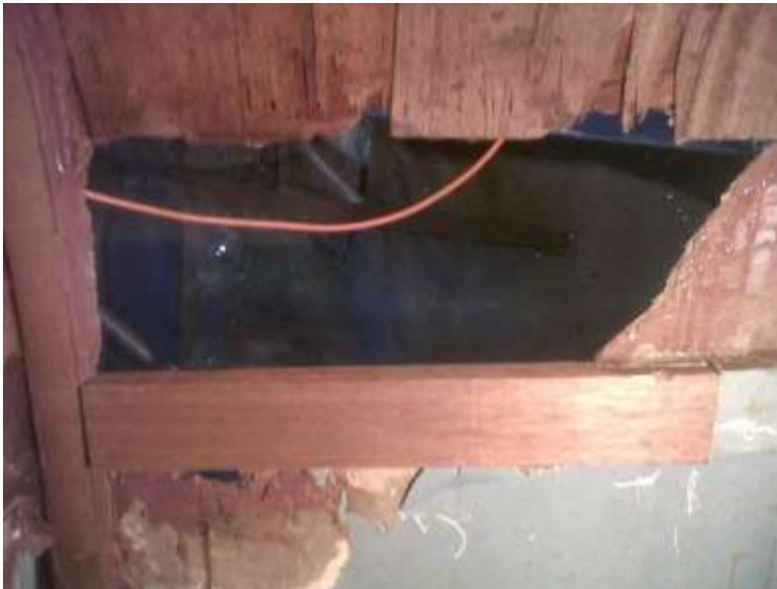
Fig 6: Strake and stringer repair
