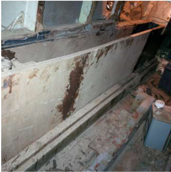
Fig 8: Keel box repairs
