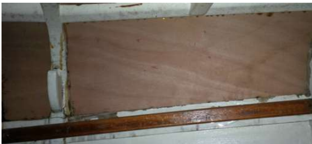
Fig 3: Aft cabin repairs
