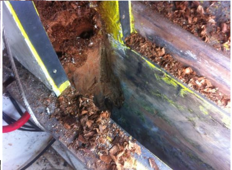
Starboard keel box end being cut out 2
