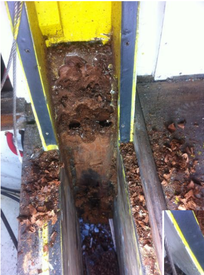
Starboard side keel box end being cut out 1
