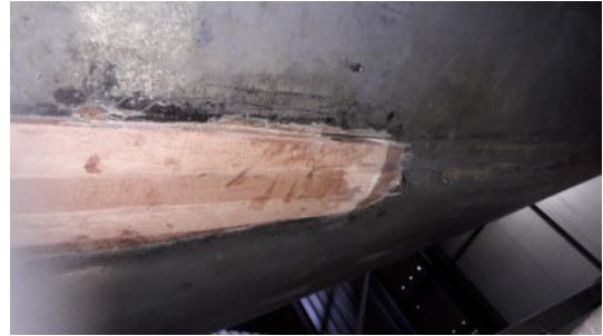
Final fairing off before coating
