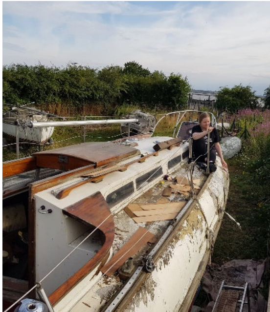
Deck repairs – 28 days and counting
