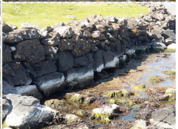
Top - One of the slipways or could it have been a noost (Shetland word for a winter refuge for a boat protected by banking), Bottom - The obvious man made stonework of the channel
