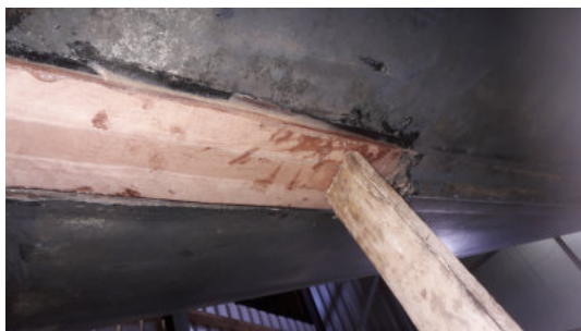
New sandkeel epoxied in place
