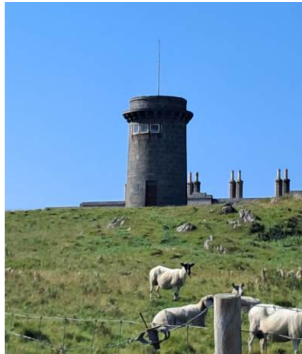
The signal tower showing the two windows facing towards the Mull, the four facing Skerrivore on the other side
