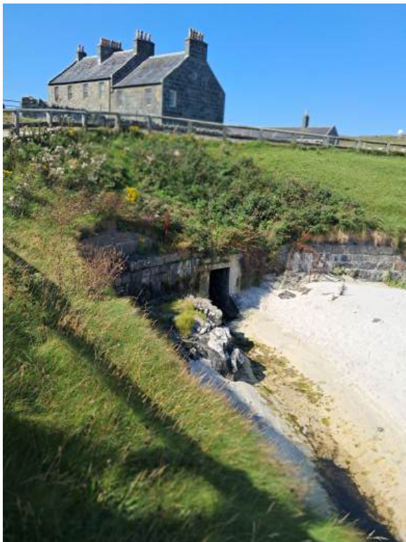
The strange culvert at the head of the harbour
