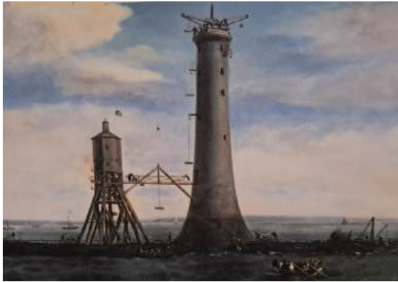
Construction of the Bell Rock lighthouse with an adjoining office / accommodation structure
