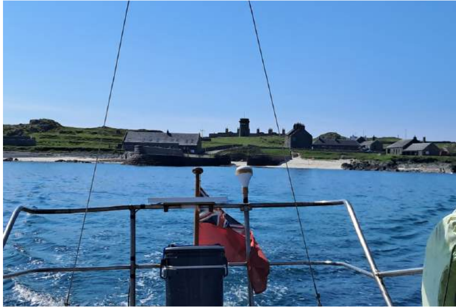
Leaving Hynish showing the pier, harbour, signal tower and the buildings all needed to run the Skerrivore Light
